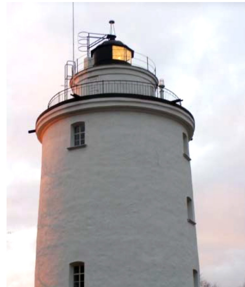
Figure 1. Suurupi lighthouse with the GNSS antenna mounted on the rooftop (Ellmann, 1997)
