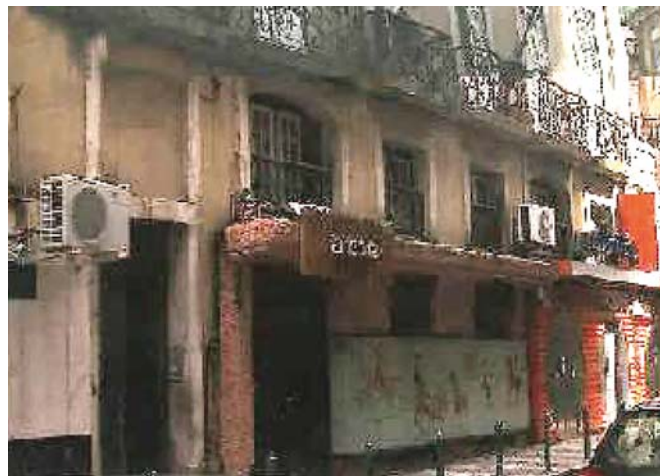
Figure 2. Condition of a building
