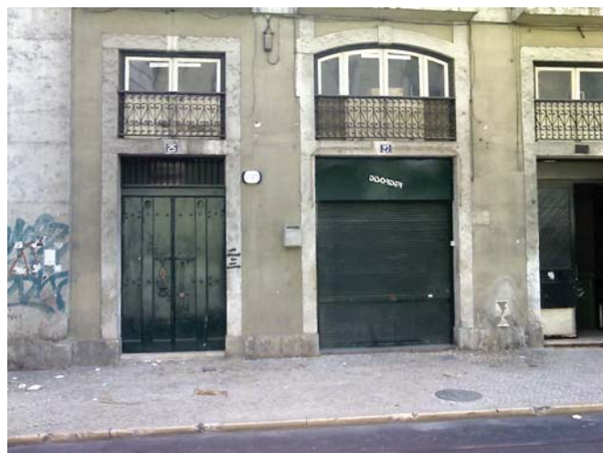
Figure 3. View of a vacant building
