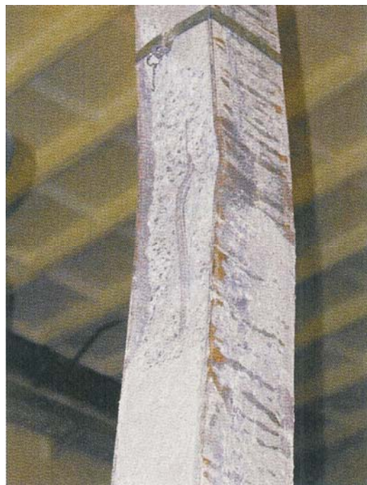
Fig. 6. Loading test of member T17 - deflection at L/2
