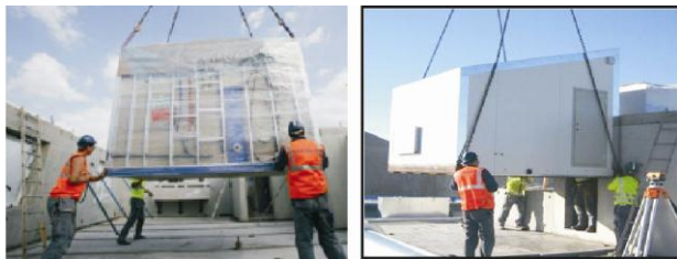
Fig. 3. Prefabricated bathroom and ventilation room modules lifted into a building site
