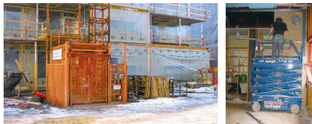
Fig. 6. Personnel, material hoist and a scissor lift
