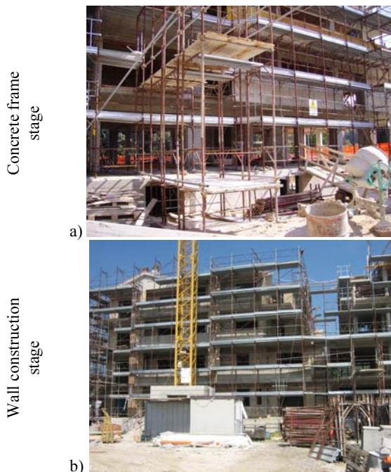
Fig. 2. Two main progress stages of the construction site
